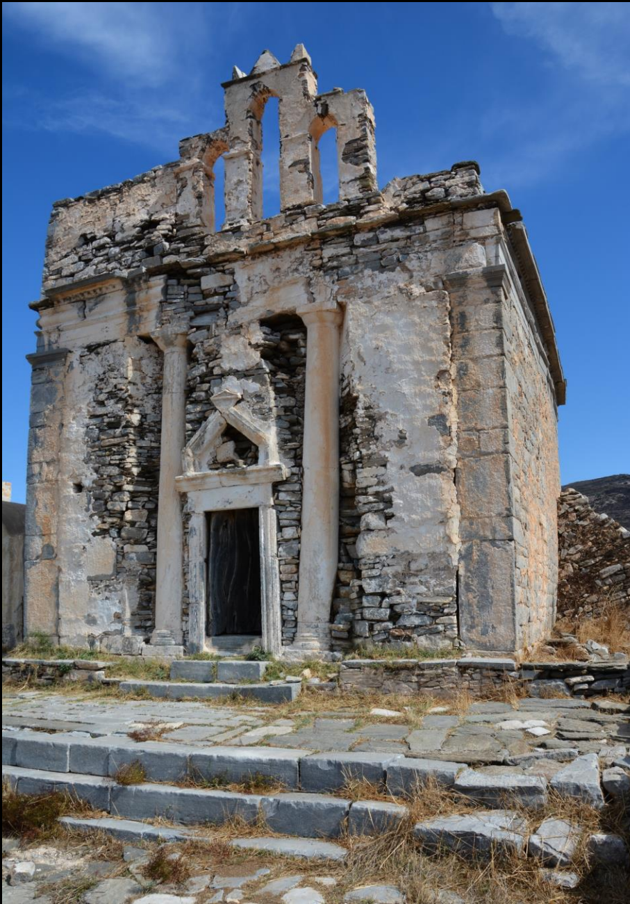
West Façade – before
