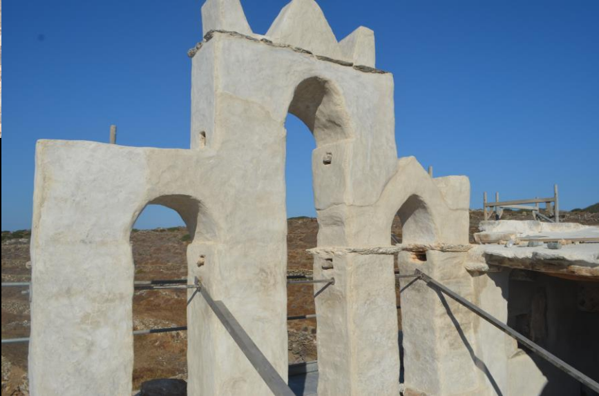
Stainless steel struts to support the belfry
