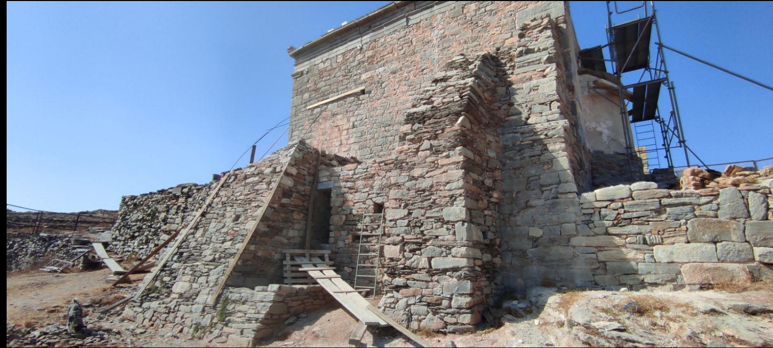
Rebuilding the medieval west buttress
